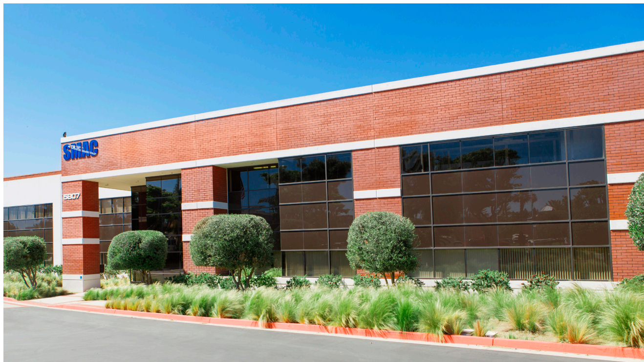
SMAC Corporate Headquarters and Factory
